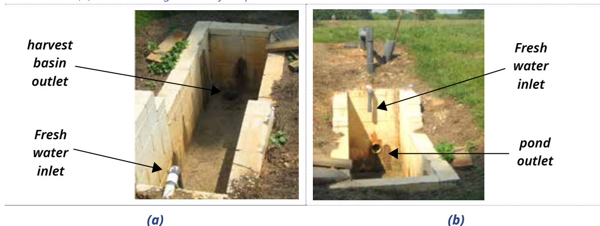
Figure 11: Harvest Basin Outside Pond. (a) View from pond wall showing outlet within harvest basin (b) View showing water inflow points into harvest basin
