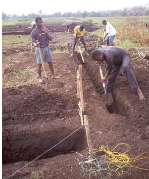
Figure 8: Constructing the Core Trench
