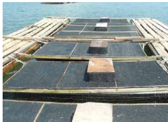
Rigid frame doubling as work platform
