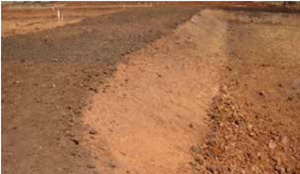
Figure 14: Finishing the Bank.
